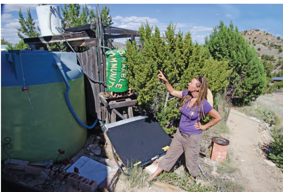
Amanda pointing to their outdoor shower, which is located next to one of the water collection tanks. The black panel serves as a solar water heater.
